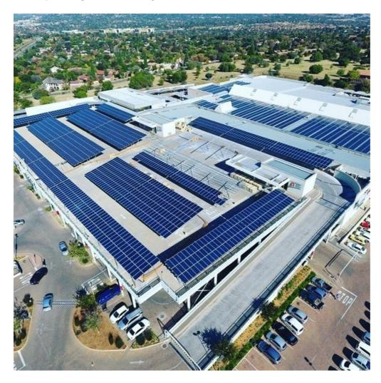
The photovoltaic (PV) solar farm, comprising 10,900 panels, produces approximately 1.2MWh of electricity. The solar farm is Emira's second solar installation and follows its successful solar power pilot project launched in 2015 at its Epson Downs Shopping Centre in Bryanston, which produces around 271kWp and saves over 515,000kWh each year.
