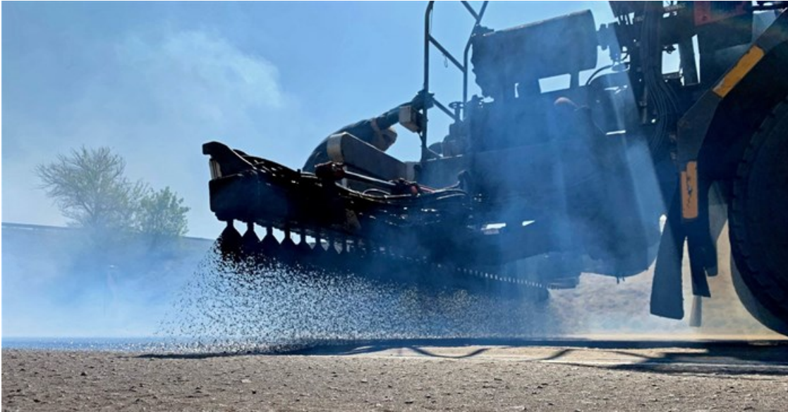
Rubber bitumen being applied for a spray seal application
