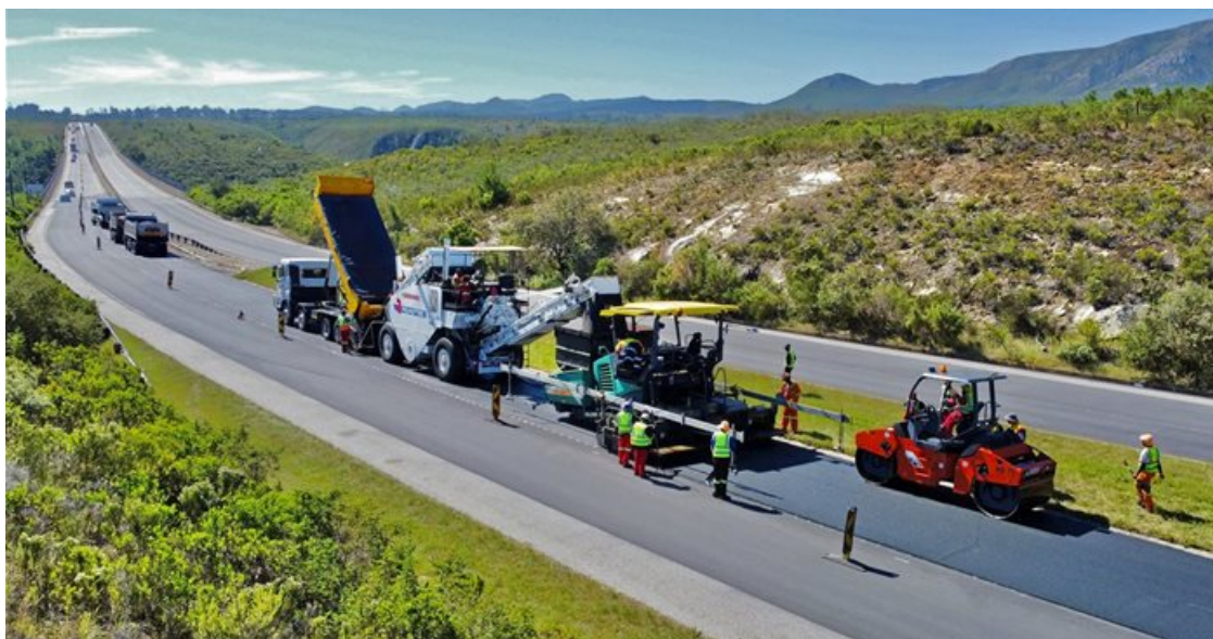
Rubber bitumen in a typical asphalt overlay application on the N2 near Garroos River.
