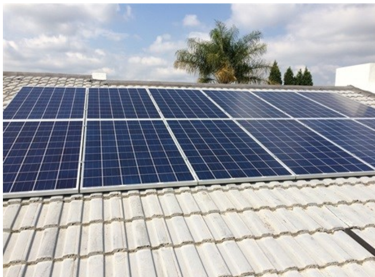
An array of 12 roof-mounted photovoltaic (PV) panels
